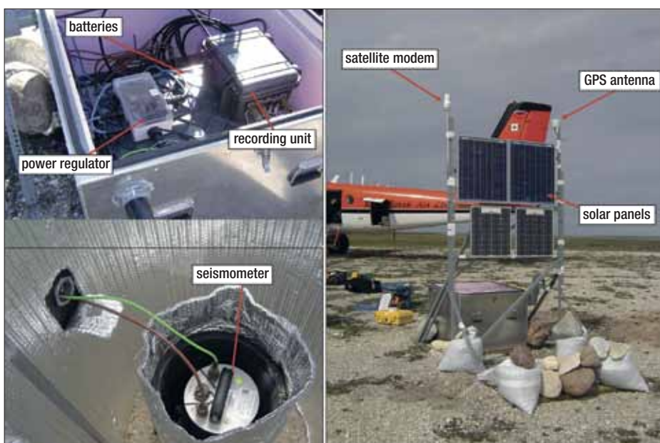
4: HuBLE-UK remote station construction. 20–40W solar panels on a steel frame recharge 3×100Ah batteries that power the seismometer and recording equipment. The GPS antenna provides continuous accurate timing information. Remote communication with the stations is via an Iridium satellite modem antenna that was scheduled to operate twice weekly. All field equipment is provided by NERC's seismic equipment pool, SEIS-UK (box 1).
